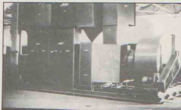
Picture shows a MVB-125.E shipped to M/s. Euphoric Drugs, capable of delivering 125000 cfm of air. Design conditions 20% RH.
