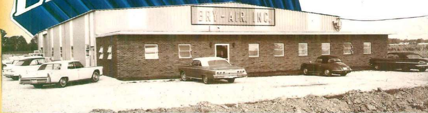
Bry-Air Plant - Fall of 1964, first phase construction
