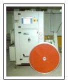
The fresh air is either precooled partially and then passed through a rotary desiccant dehumidifier, where the moisture content is reduced to the desired level. This air is passed over a heat exchanger coil fed with a cooling tower
