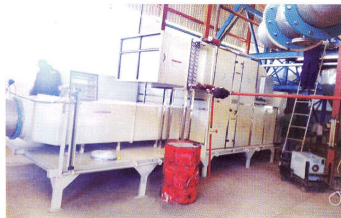
Figure 3: Skid mounted integrated dehumidification system
