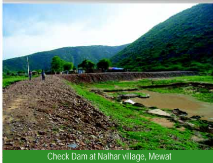
Check Dam at Nalhar village, Mewat
