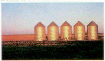
When material is stored in silos, generally it is not filled up to the top, but some space is left empty for air circulation. This empty space creates it's own problem as moisture builds up in the unfilled portion. Due to variation of temperaure outside the silos, condensation of water vapour takes place inside the silos leading to:
